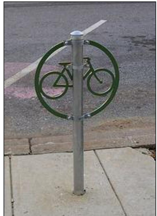
Figure 3.3 – Ring & Post rack directly buried in the ground
