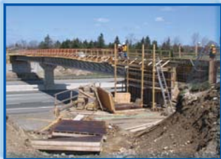
April 2007 Forming end wall at Morningside Drive
