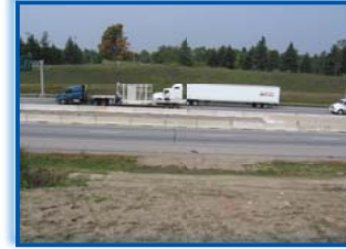
September 2005 Start of Construction
