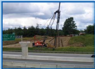
July 2006 Pile Driving Kitchener Side
