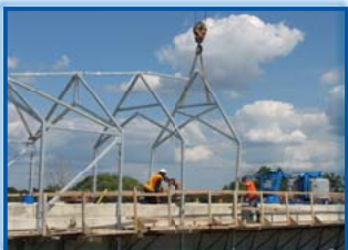
August 2007 First canopy frame is erected
