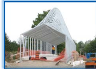
September 2007 Canopy frame arch completed
