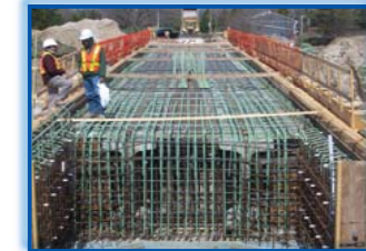
April 2007 End View-placing re-bar for concrete deck
