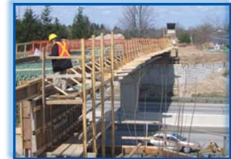
April 2007 Inspecting the bridge forming
