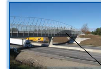
October 2007 Shadow arch installation
