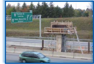
November 2005 Construction of Centre Pier
