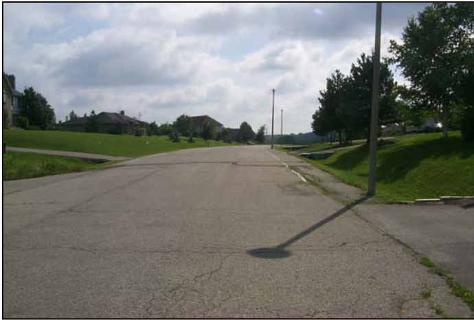
Photograph C1 Location 1: Ratcliffe Road looking east
