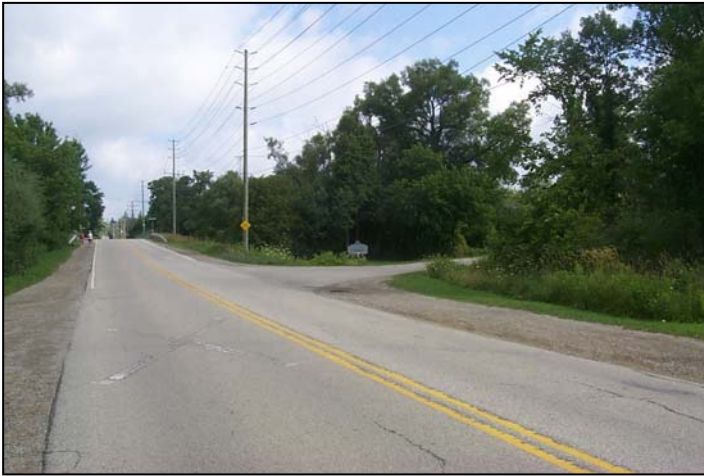
Photograph C5 Location 4: Mill Run Trail entry along Beavertdale Road
