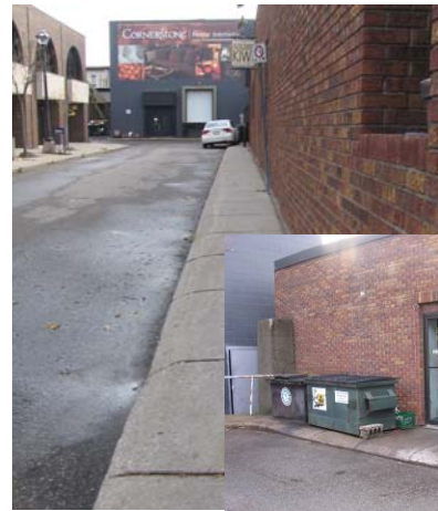
Narrow Sidewalk and Lack of Space for Large Refuse Containers on Petty Place
