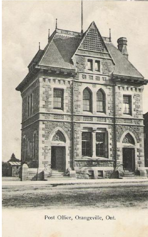
Figure 4 Postcard image of the demolished Orangeville Post Office and Customs House (Author's Collection)
