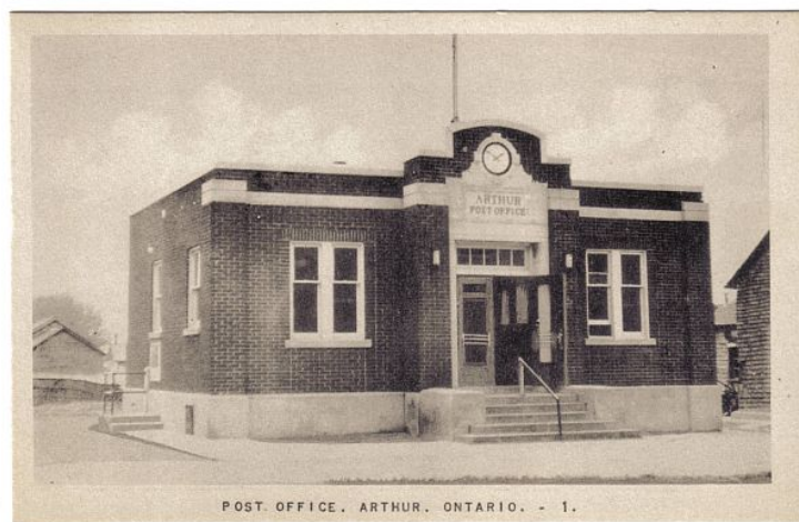
Figure 6 Postcard image of the demolished Arthur Post Office. (Author's Collection)
