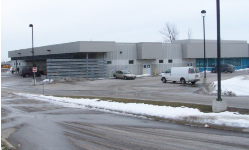
Figure 9 Photograph of Guelph Distribution Centre. (by Author)
