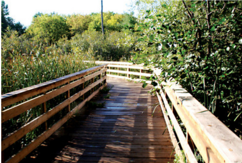
Fresh start for Riverside walk. Work at the south end of the new boardwalk has been completed and could be open to the public in the next few weeks. Ray Martin, Times Staff
