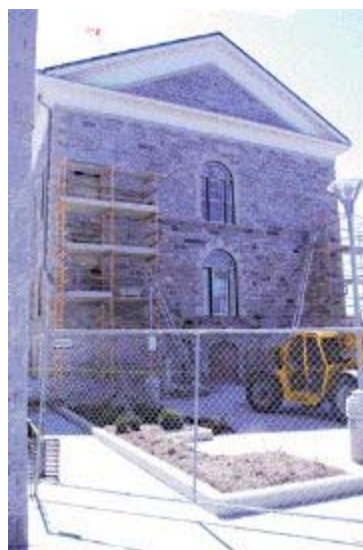
Work at historic city hall
