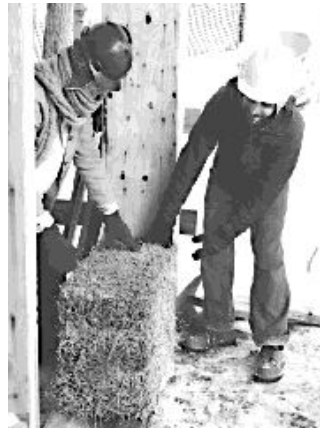
Last Friday, Chantal Cornu (left), executive director of the Grand House Student Co-op, and promotions co-ordinator Earl Beadle place the first straw bales inside the wall frames of the student housing project.
