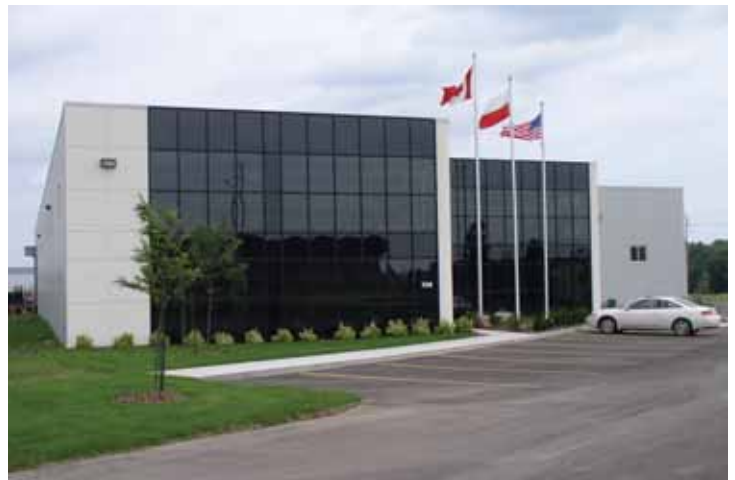
Eclipse Automation’s location at 130 Thompson Drive is currently undergoing a 27,000 square foot expansion scheduled to open in October.
