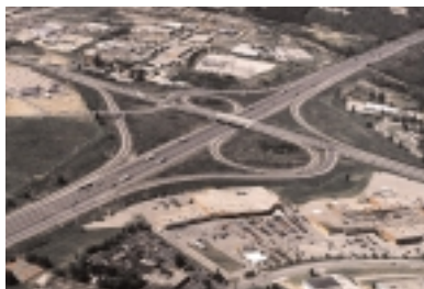
Cambridge Highway 24 and Highway 401 interchange.
